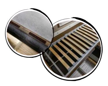
ANTI-CONDENSATION PANELS spaced away from the wall in living and sleeping areas PERIMETER HEATING in models with twin beds.
